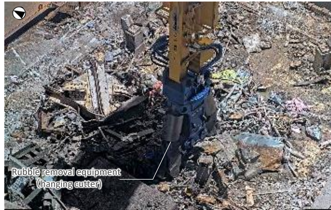
Crushing rubble on the operating floor (photographed on July 16, 2026)
