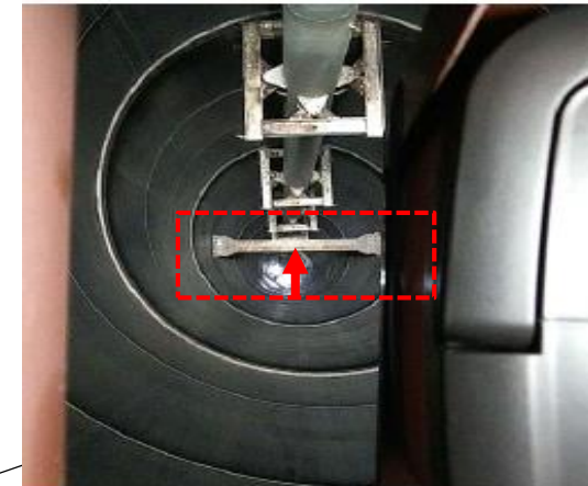
Steel frame inside the stack (shown from above)
