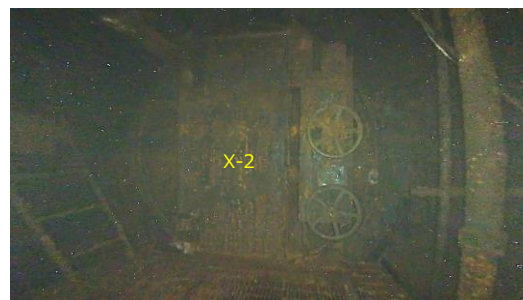
① : X-2 penetration
