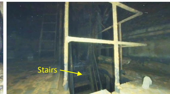
④ : Subfloor stairs (north)
