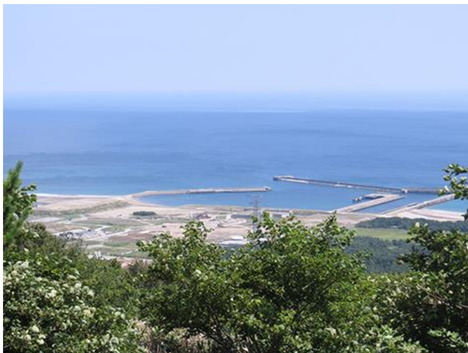
Planned construction site of the Higashidori Nuclear Power Station
