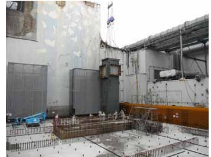
First column installation complete
