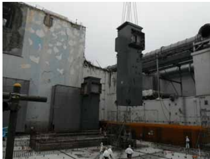
Second column being installed
