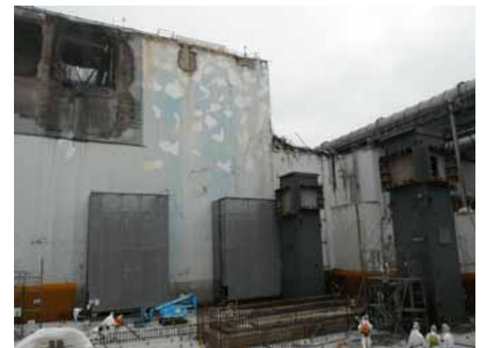
Second column installation complete
