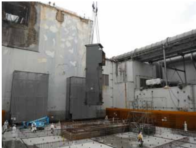
First column being installed
