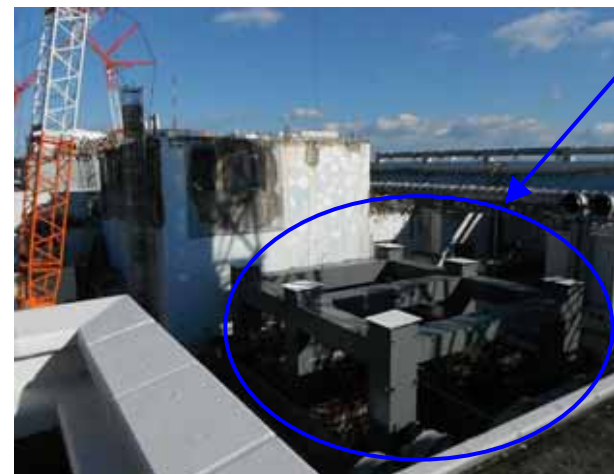
Cover being constructed for fuel removal at Unit 4
