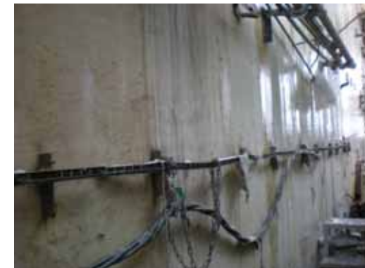
10 SFP side wall (West side)
