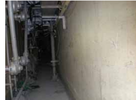
8 SFP side wall (South side)
