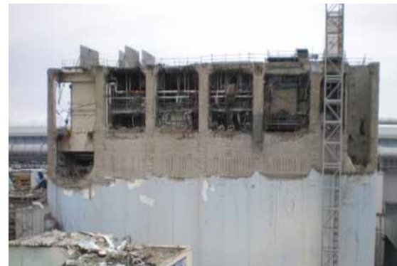
⑤ West wall (Outer wall)
