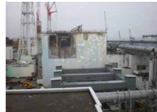
⑥ South wall (Outer wall)
