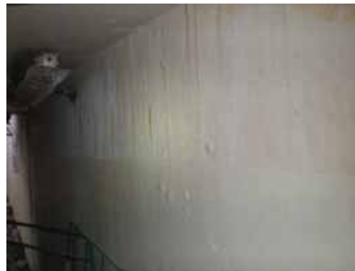
9 SFP side wall (East side)
