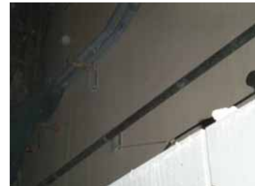
④ West wall (Inner wall)
