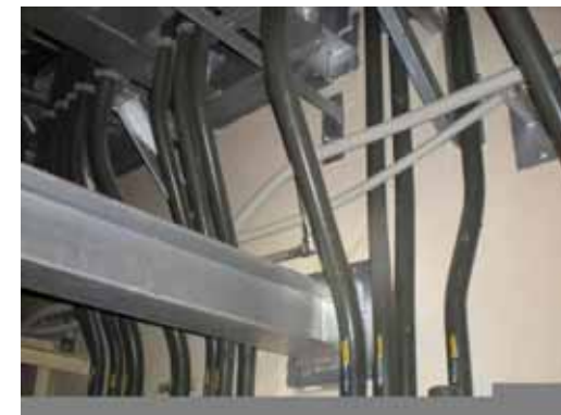
② South wall
