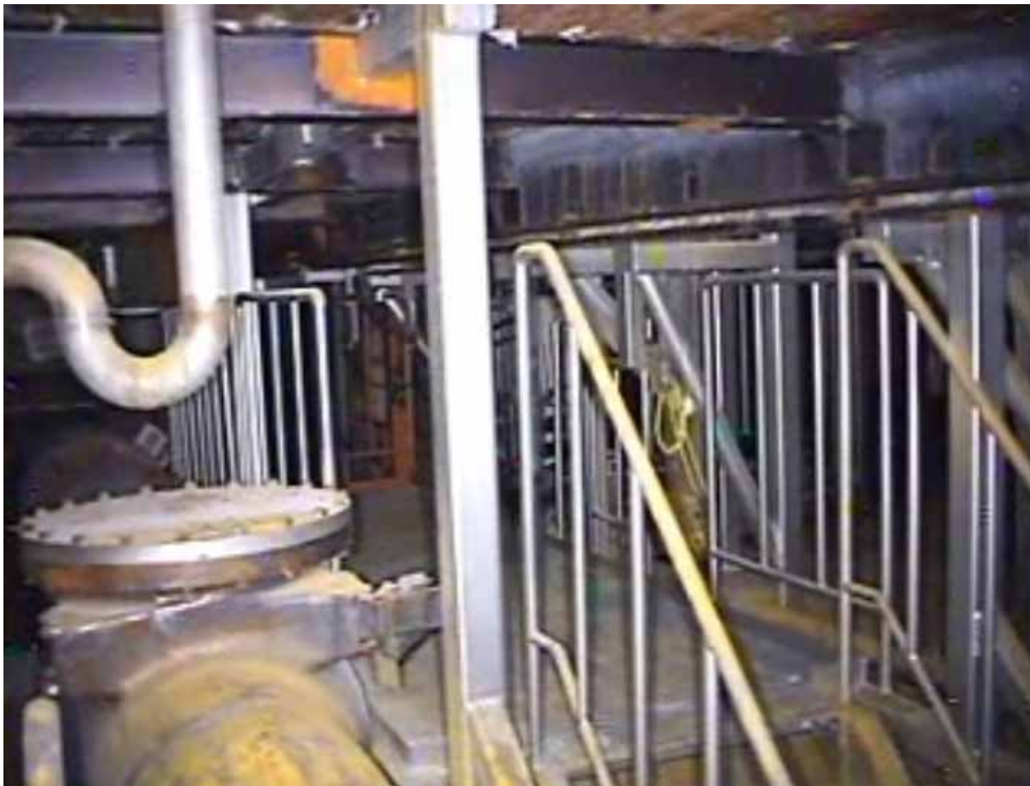
Photo taken on February 20, 2013 by TEPCO
