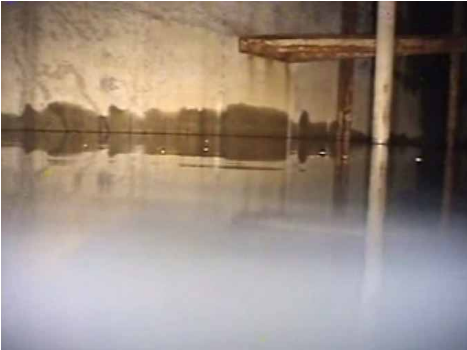
Photo taken on February 20, 2013 by TEPCO
