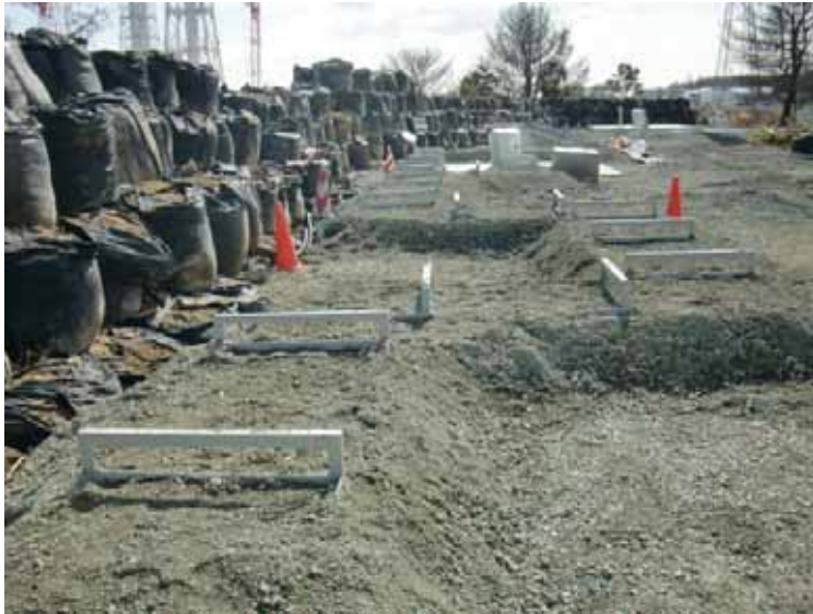
Foundation installation for A system piping
