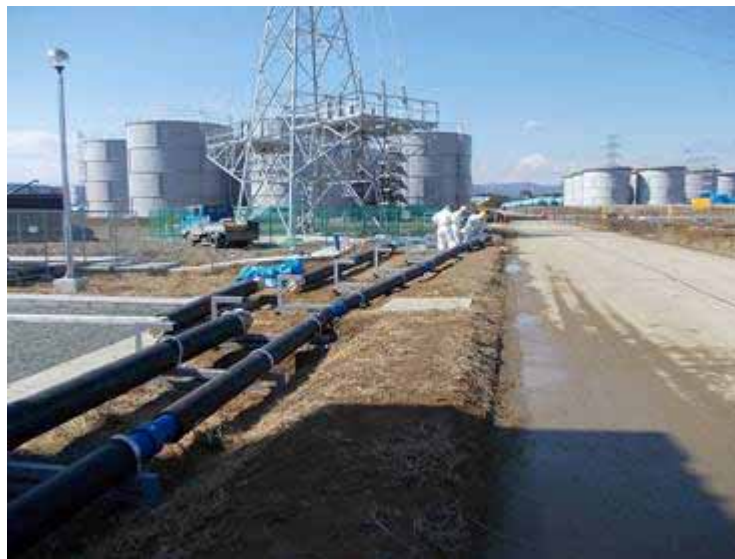
Transfer pipes from each system to the temporary storage tank
