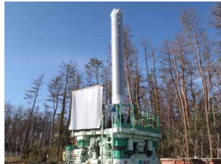
Inner pipe installation for pump well No.10 (B system)
