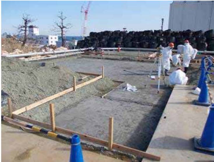
A system buffer tank installation
