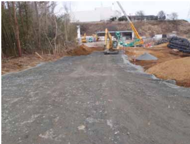
Yard development for pump wells No.7-8 (B system)
