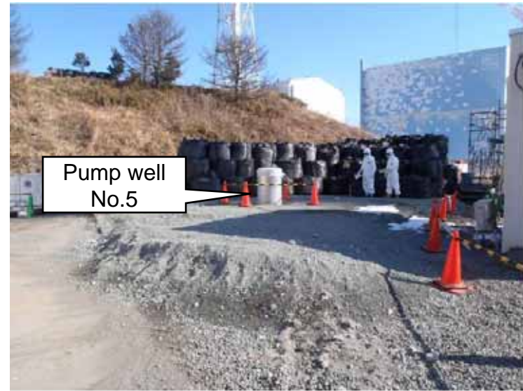
Drilling completed for pump well No.5 (B system)
