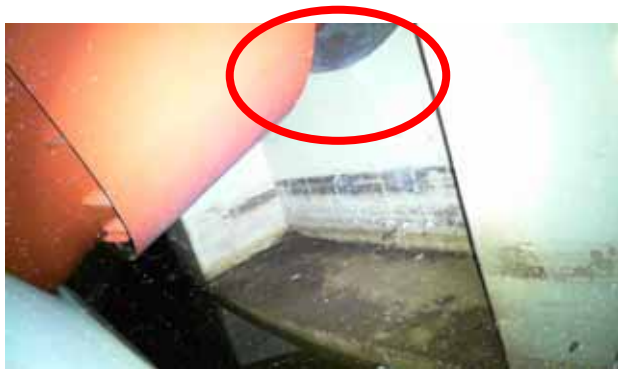
Edge of the vent pipe sleeve
