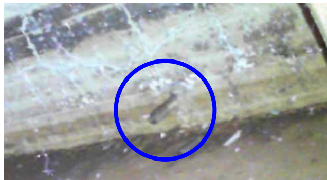
Edge of the sand cushion drain pipe
