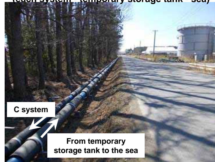
Transfer pipe installation (C system, temporary storage tank - sea)
