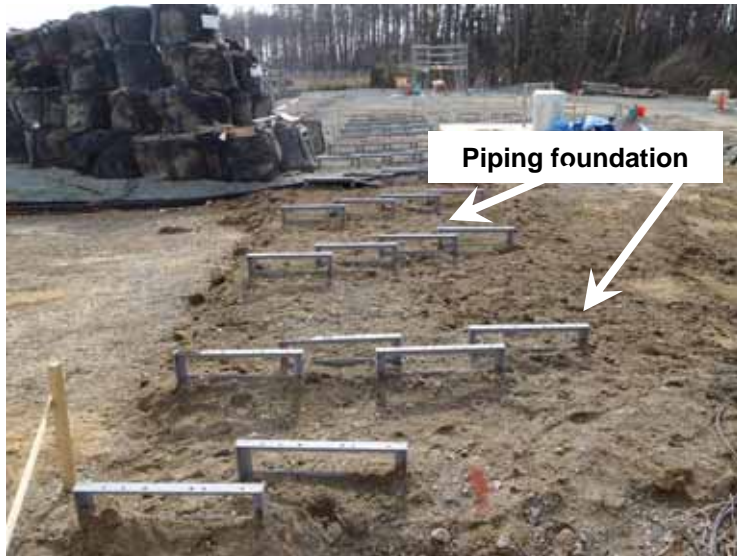
Foundation installation for piping (B system)
