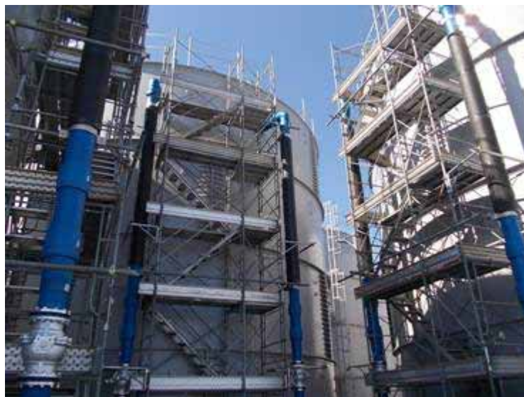
Temporary storage tank installation
