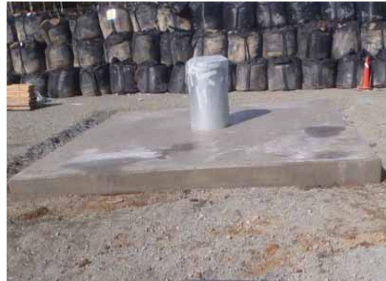
Installation of pump well No.9 (B system) completed
