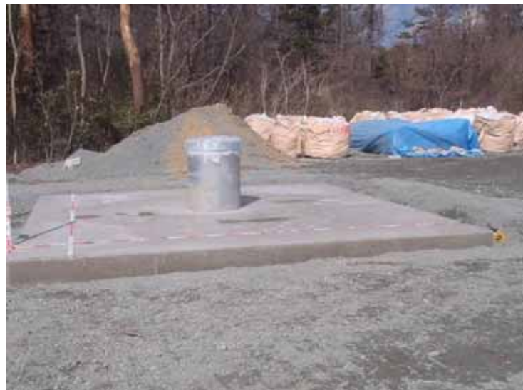
Installation of pump well No.11 (system C) completed
