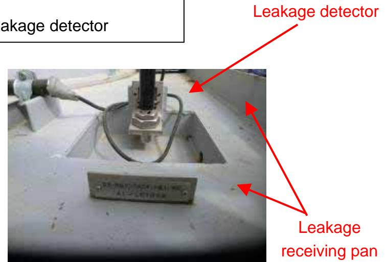
(Example) Leakage detector installed in the equipment skid
