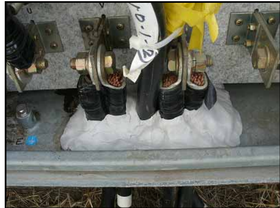
After seal was applied
