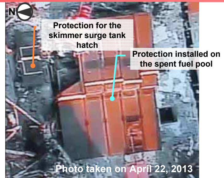
Before the protection on the spent fuel pool was renewed
