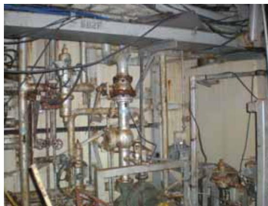
⑥ SFP side wall (East side)
