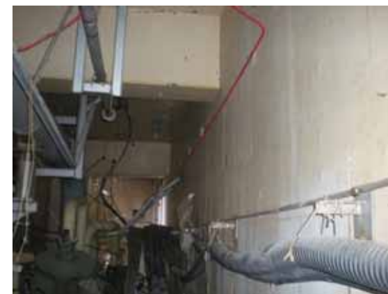
⑨ SFP side wall (West side)
