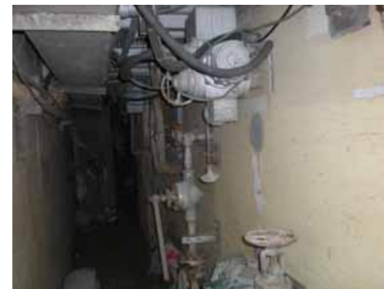
⑦ SFP side wall (South side)
