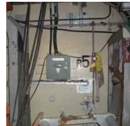
④ West wall (Inner surface)
