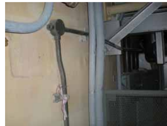
② South wall
