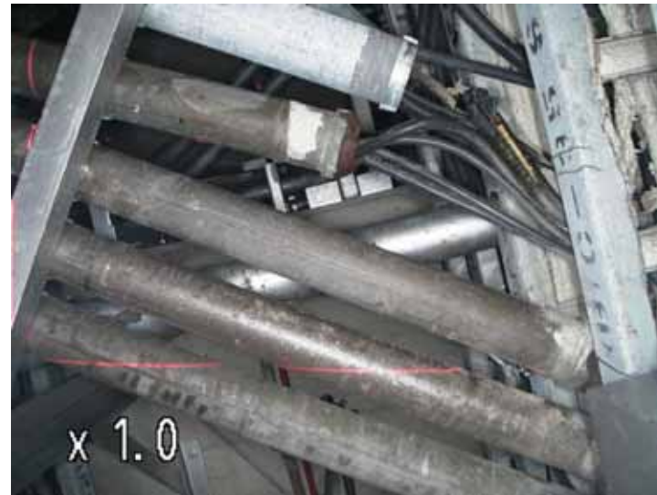
Picture point (1): Conditions of the ceiling
