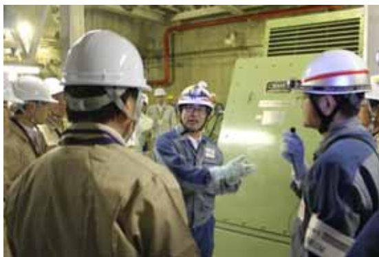
Emergency diesel generator (generator) (in the 2 nd basement of the Reactor Building Annex)
