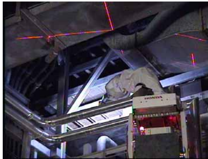
(5) Stop position of the high-access survey robot [1]
