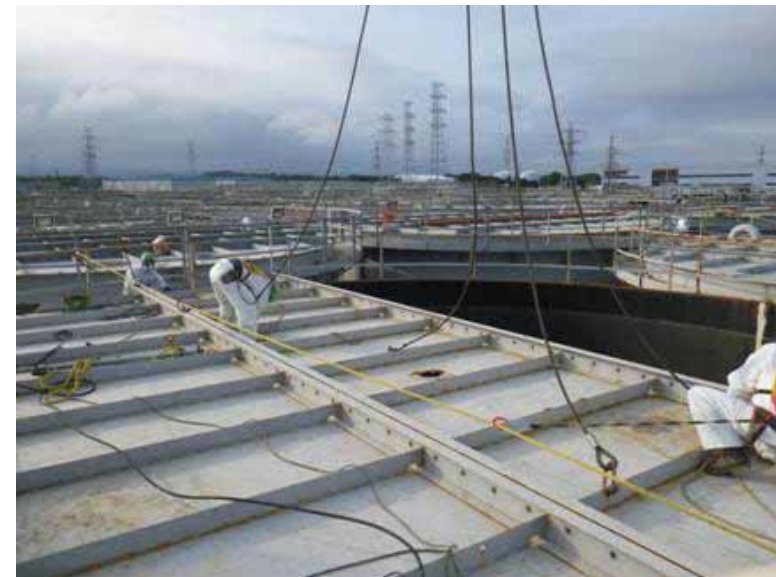
Top plates removal
