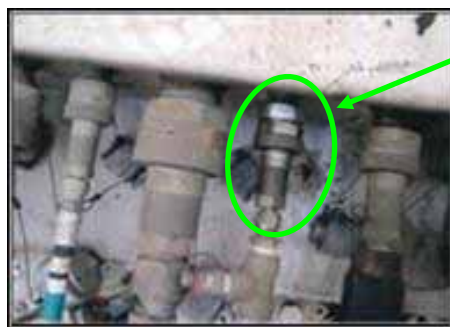
The assembly/disassembly screw joint
