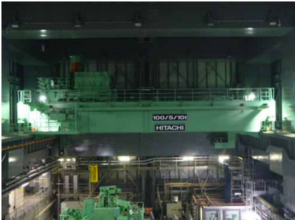
Source: Photo taken by TEPCO on September 19, 2013
