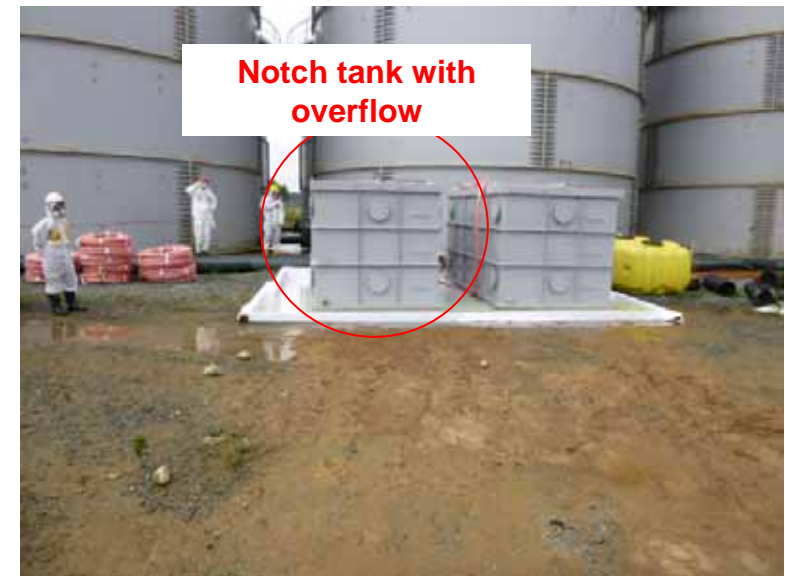
Photo taken by TEPCO on October 1, 2013
