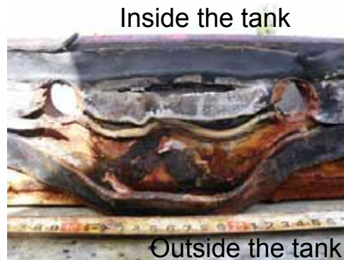
Under removal (Bottom plate B)
