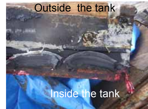
Under removal (Side-plate side near ②)
