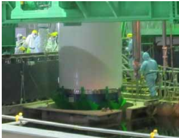
Bringing the container down to the pool water (1)
