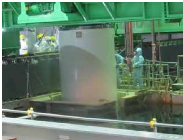
Bringing the container down to the pool water (2)
