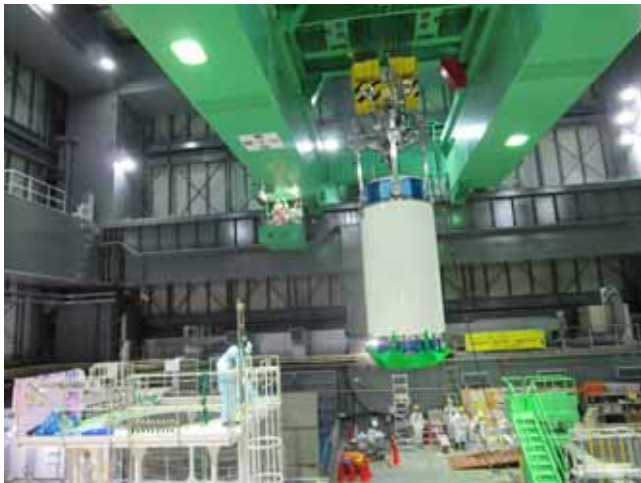
Lifting up the on-premise transportation container (1)
