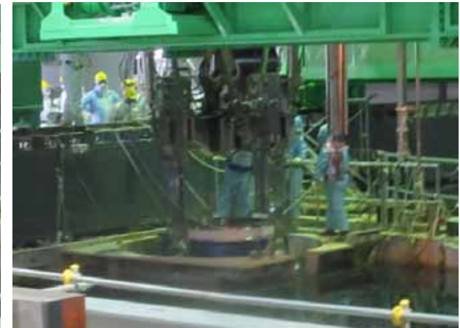
Bringing the container down to the pool water (3)
