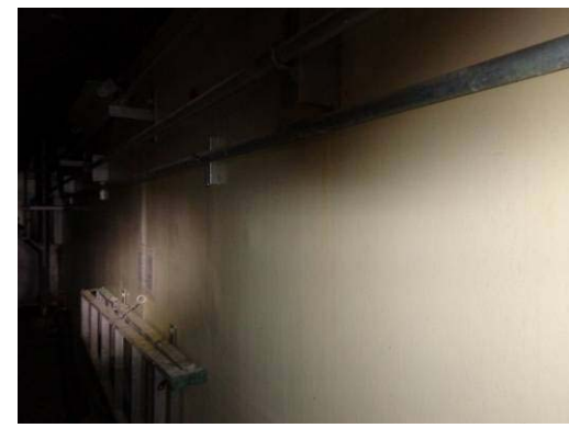
④ West wall (inner surface)
