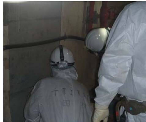
Visual inspection at a turbine building
