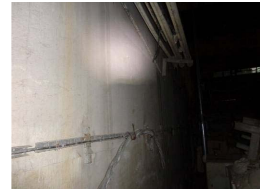
⑨ SFP side wall (West side)
