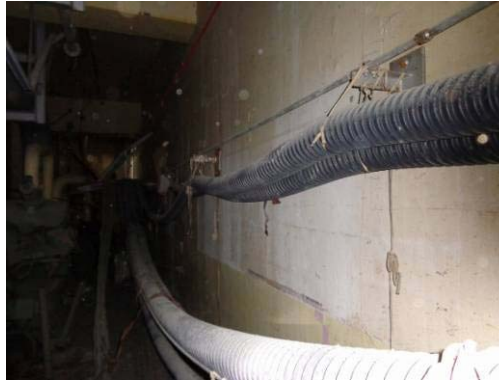
⑥ SFP side wall (East side)
