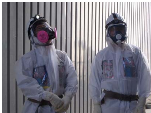
Visual inspection for South outer wall
