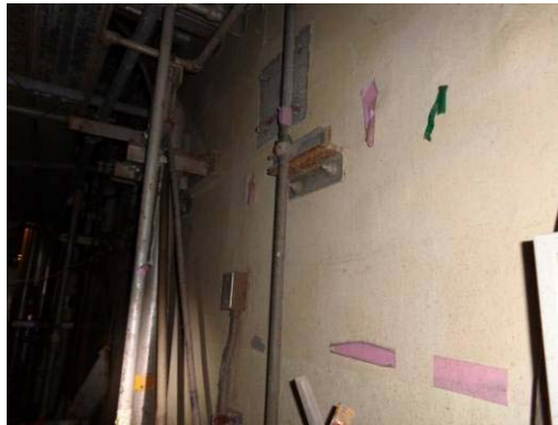
① West wall (inner surface)
