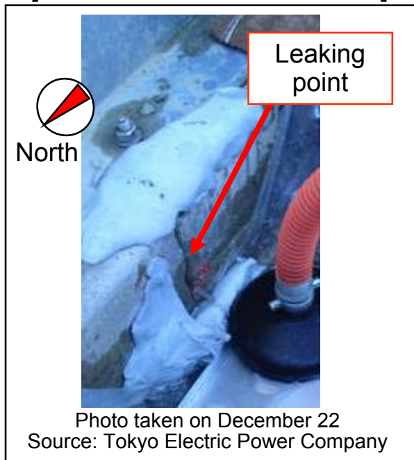
[West dike at H5 tank area]
