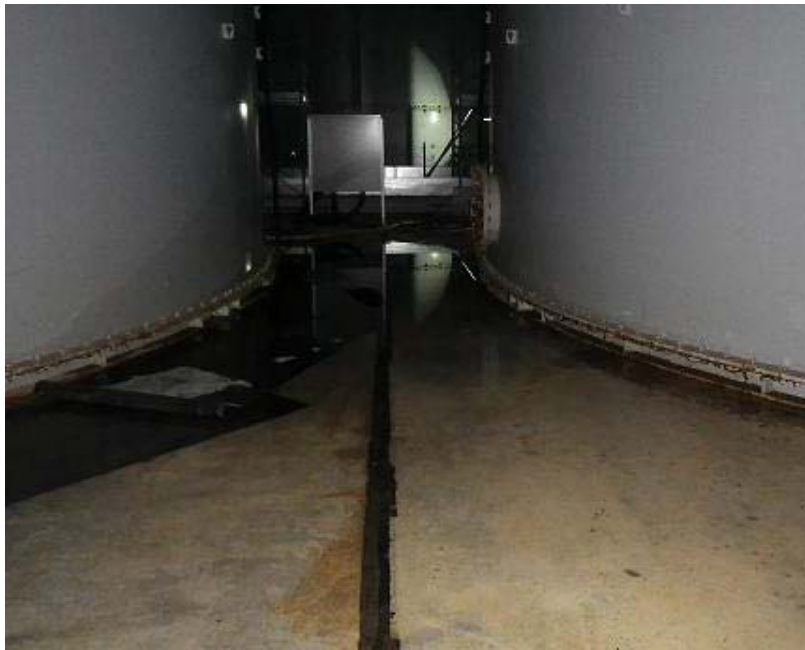
Condition of the concrete casting joint (H4 East area)
