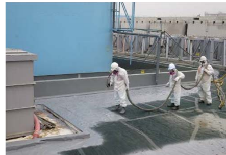
Coating works inside the dike
