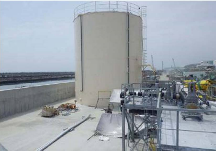
Water collecting tank installation
