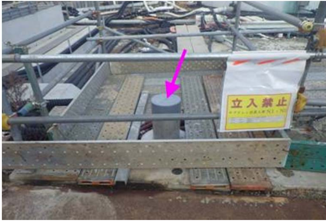
Newly installed subdrain pit N1 (excavation completed)
