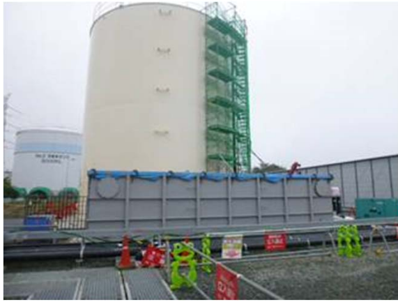
Sampling tank installation
