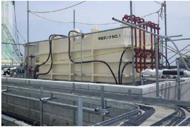
No 1 relaying tank installation
