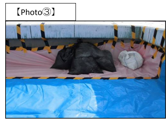
Blue sheet placing work
