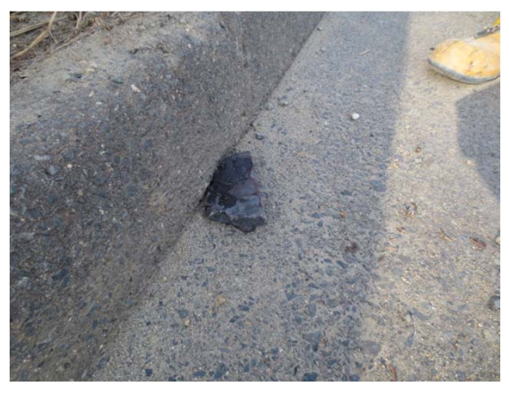
Scene of fire (on the road③)
