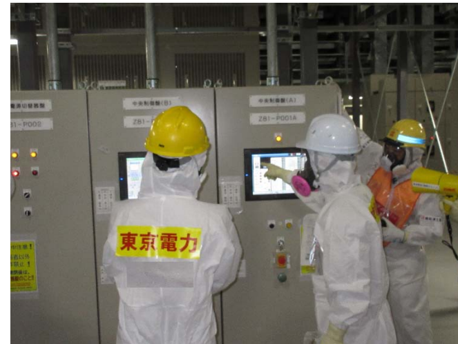
Final check before start-up
