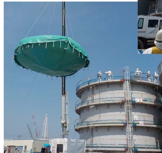
←Setting up temporary top board
