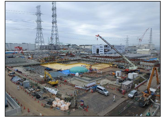
After dismantling (photo taken on October 29)
