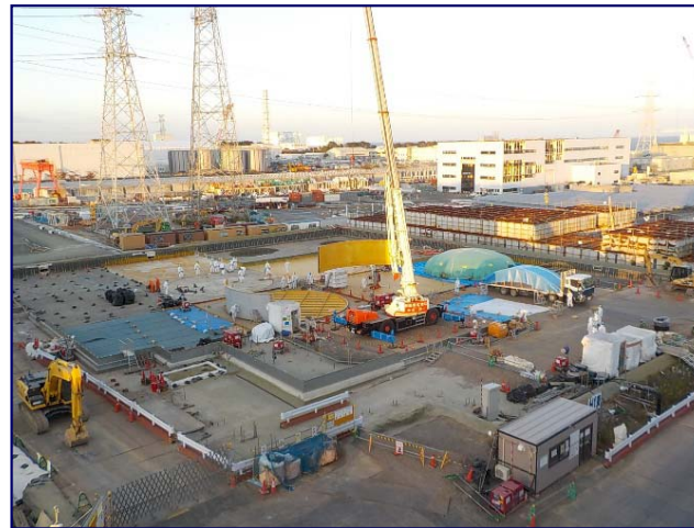
During dismantling (photo taken on October 28)
