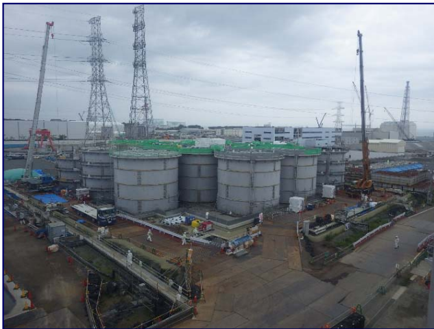
Start of dismantling (photo taken on June 19)
