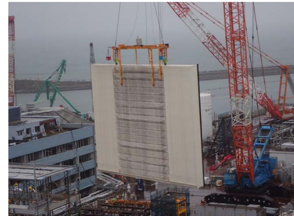
Wall Panel Taken Down (Expanded)
