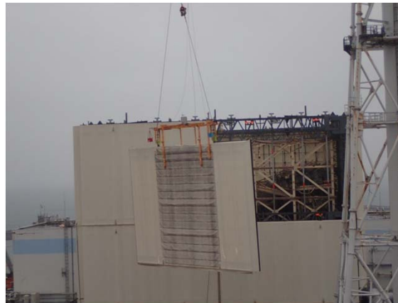
Wall Panel Opened (Expanded)
