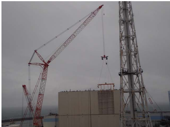
Before Wall Panel Lifted Up (Full View)
