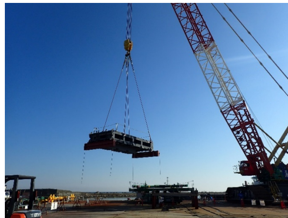
Being lifted by a crane from a barge
