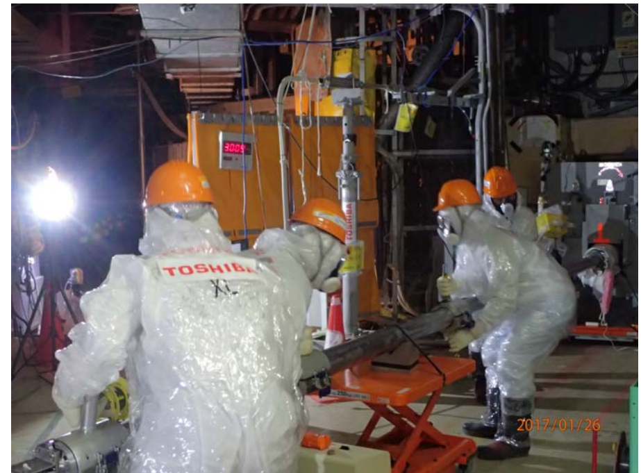
Inside of Unit 2 Reactor Building
