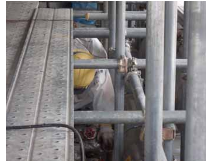
Refrigeration valve opening work
