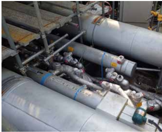
Condition of freezing pipes and valves
