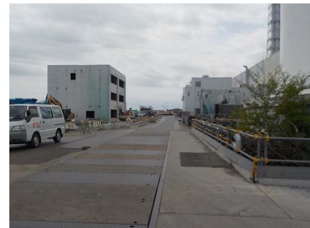
Sea-side road of Unit 3
