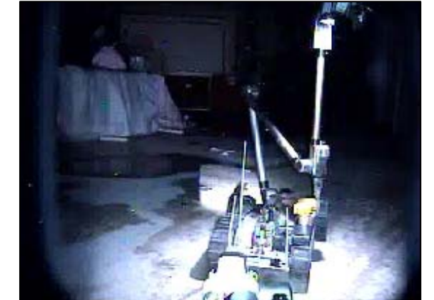
②Around Airlock (North), R/B dose 68.2mSv/h , temp 30.2°C humidity 44.0% , O2 20.9%
