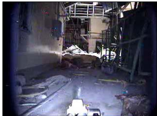
⑩West side corridor dose 120.0mSv/h , temp 28.6°C humidity 36.4% , O2 20.9%
