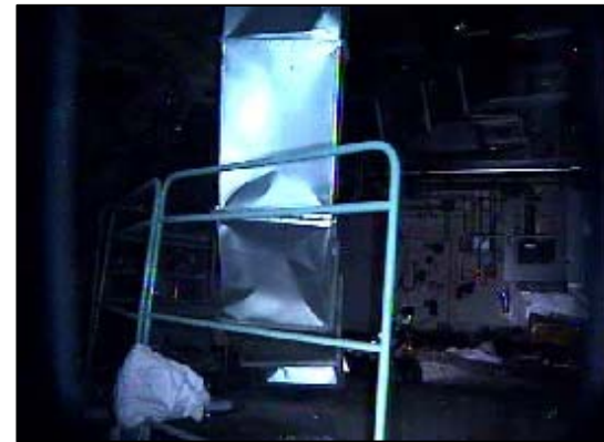
⑧Hydraulic Control Unit~Airlock (West) dose 63.7mSv/h , temp 28.5°C humidity 38.3% , O2 20.9%
