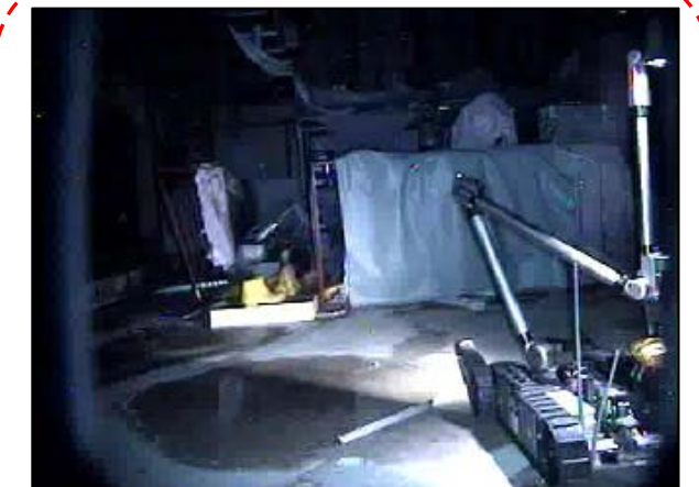
③Around Airlock (North), R/B dose 48.6mSv/h , temp 30.4°C humidity 43.6% , O2 20.9%
