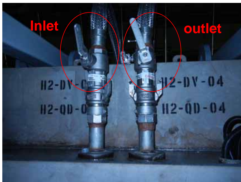
Joints of cesium adsorption tower
