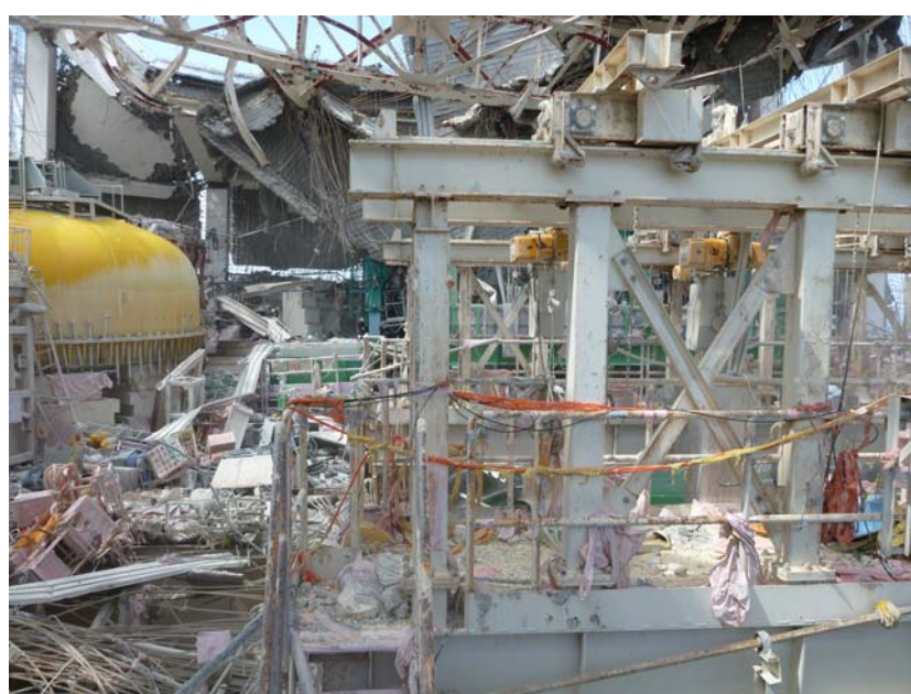
Equipment Storage Pool side to the Fuel Exchange Truck
