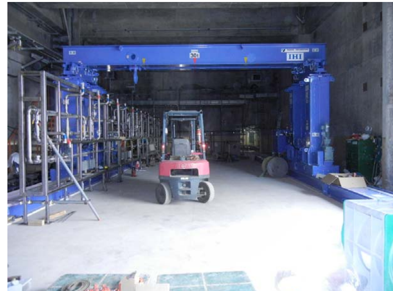
Installing a lifting equipment for changing containers
