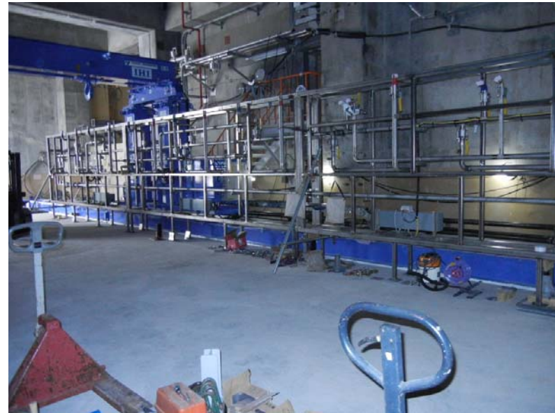
Installing valves and piping
