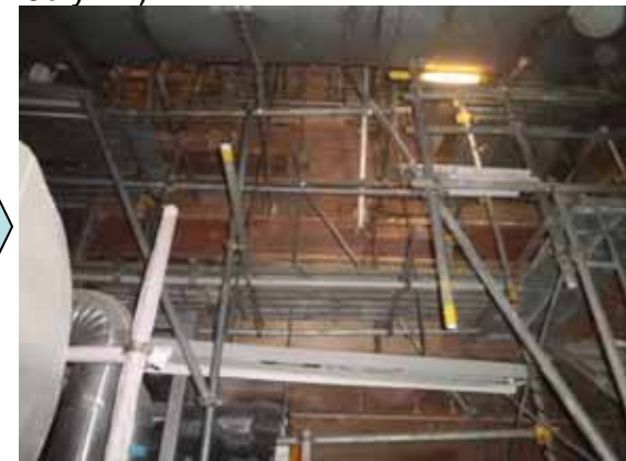
Completion of installation of supporting structure (Pictured on July 30)
