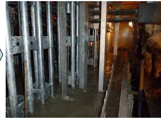
Concrete placement (pictured on July 21)
