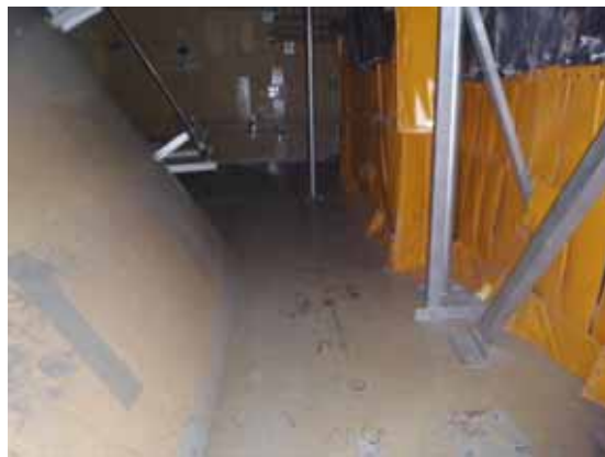
Before installation of the steel support pillars (pictured on May 31)
