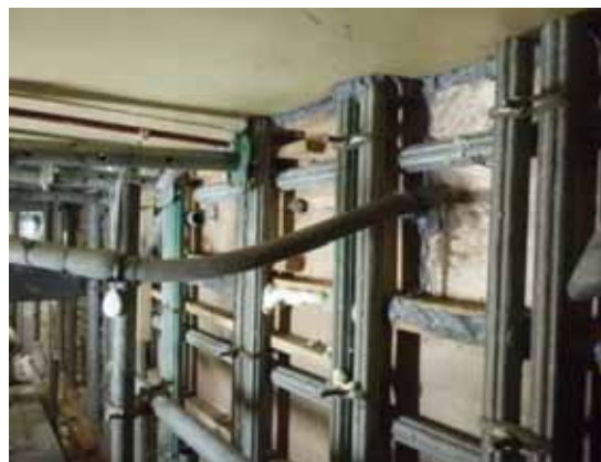
Injection of grouting (pictured on July 30)
