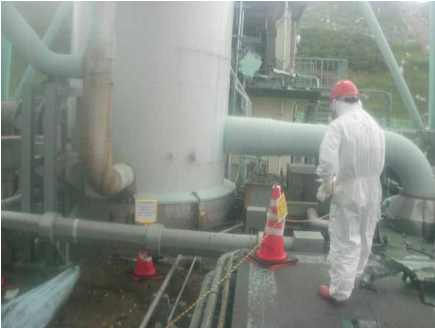
Photo taken at stack drain pipe of exhaust stack of Units 1 and 2 taken around 3:30 pm on August 4, 2011 taken by Tokyo Electric Power Company
