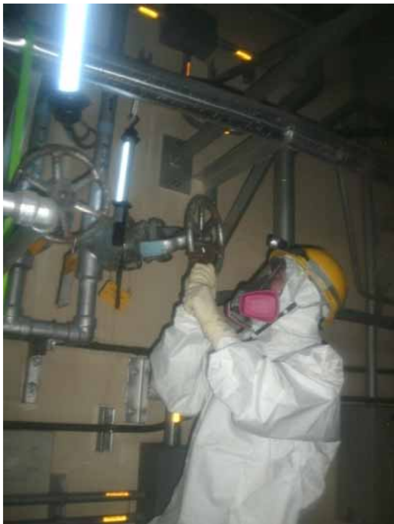
Lineup of Make-up water system and valve operations
