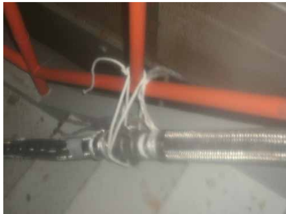
Installation of flexible hose pipe
