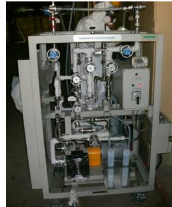
Fukushima Daiichi: Temporary gas sampling instrument for primary containment vessel (PCV) of Unit 1
