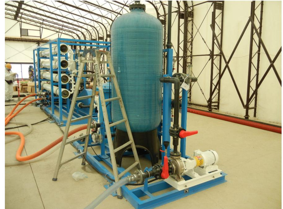
Water Desalinations (filtering apparatus)
