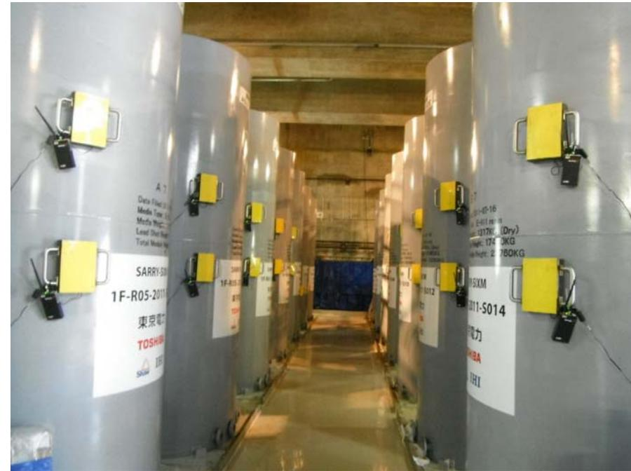
2nd Cesium adsorption apparatus No2
