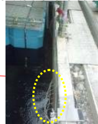
⑤ Wire mesh, inlet of the air-conditioning at Spent Fuel Pool was bent to the reverse direction
