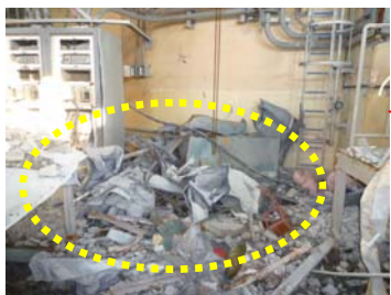
⑦ Rubbles from air-conditioning ducts
