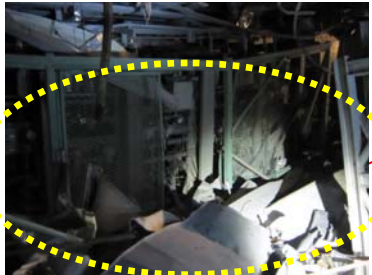
⑭ Floor pushed down (in front is rubbles from air-conditioning ducts)
