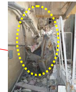
⑪ Rubbles from air-conditioning ducts (no air-conditioning ducts above)
