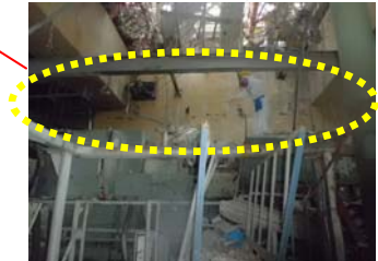
⑫ The original place of installation of air-conditioning ducts
