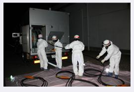
At the time of all AC power loss, to maintain functions of water injection and heat removal for the reactors, Spent Fuel Pools, we conducted a training by utilizing a power source car aimed at supplying sufficient power.
