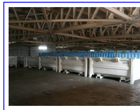
• Temporarily placed debris container
